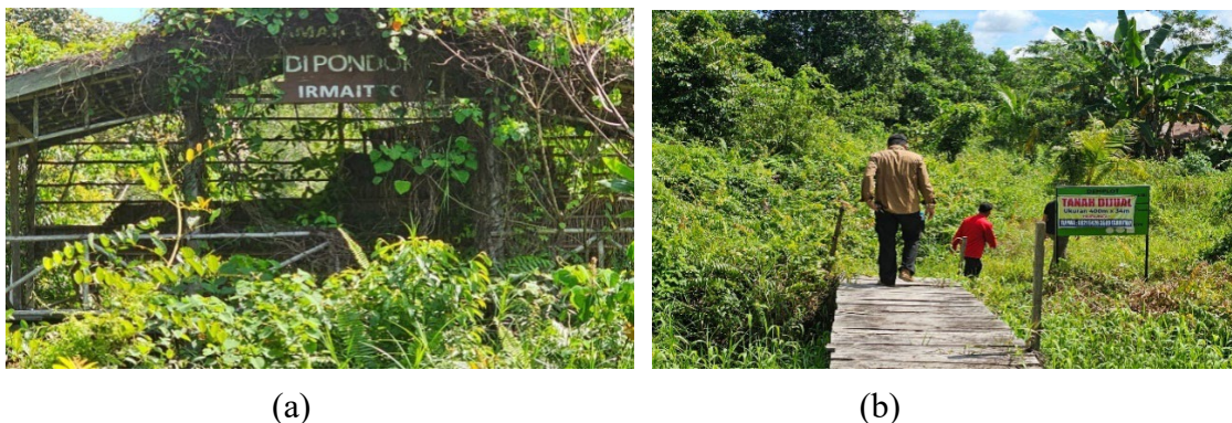
Figure 4. Abandoned and degraded shelter for workers (a); land is advertised for sale (b)
